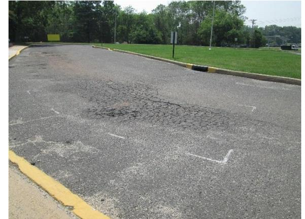
The parking lot is very eroded. Parking spaces can be replaced with pervious pavement to collect and infiltrate runoff. Two rain gardens can also be installed capture, treat, and infiltrate driveway runoff. A preliminary soil assessment suggests that more soil testing would be required before determining the soil's suitability for green infrastructure
