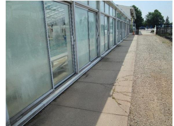
There is a sidewalk along the enclosed pool that is severely eroded, and can be replaced with pervious pavement to allow water to infiltrate. Rain gardens can also be installed to capture, treat, and infiltrate roof runoff. A preliminary soil assessment suggests that the soils have suitable drainage characteristics for green infrastructure.
