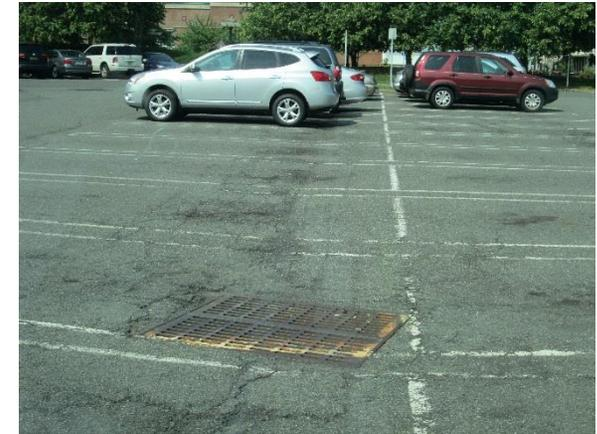
Along the east side of the mall, near the Lord & Taylor department store, pavement is eroded around existing catch basins. Parking spaces can be replaced with pervious pavement collect and infiltrate runoff before it reaches these catch basins. A preliminary soil assessment suggests that more soil testing would be required before determining the soil's suitability for green infrastructure.
